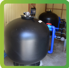
Improved filtration system with UV sterilizer
